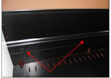
Look inside and take note of how the runners are fitted to the drawer, there is a front and rear tag lancing on each side.
